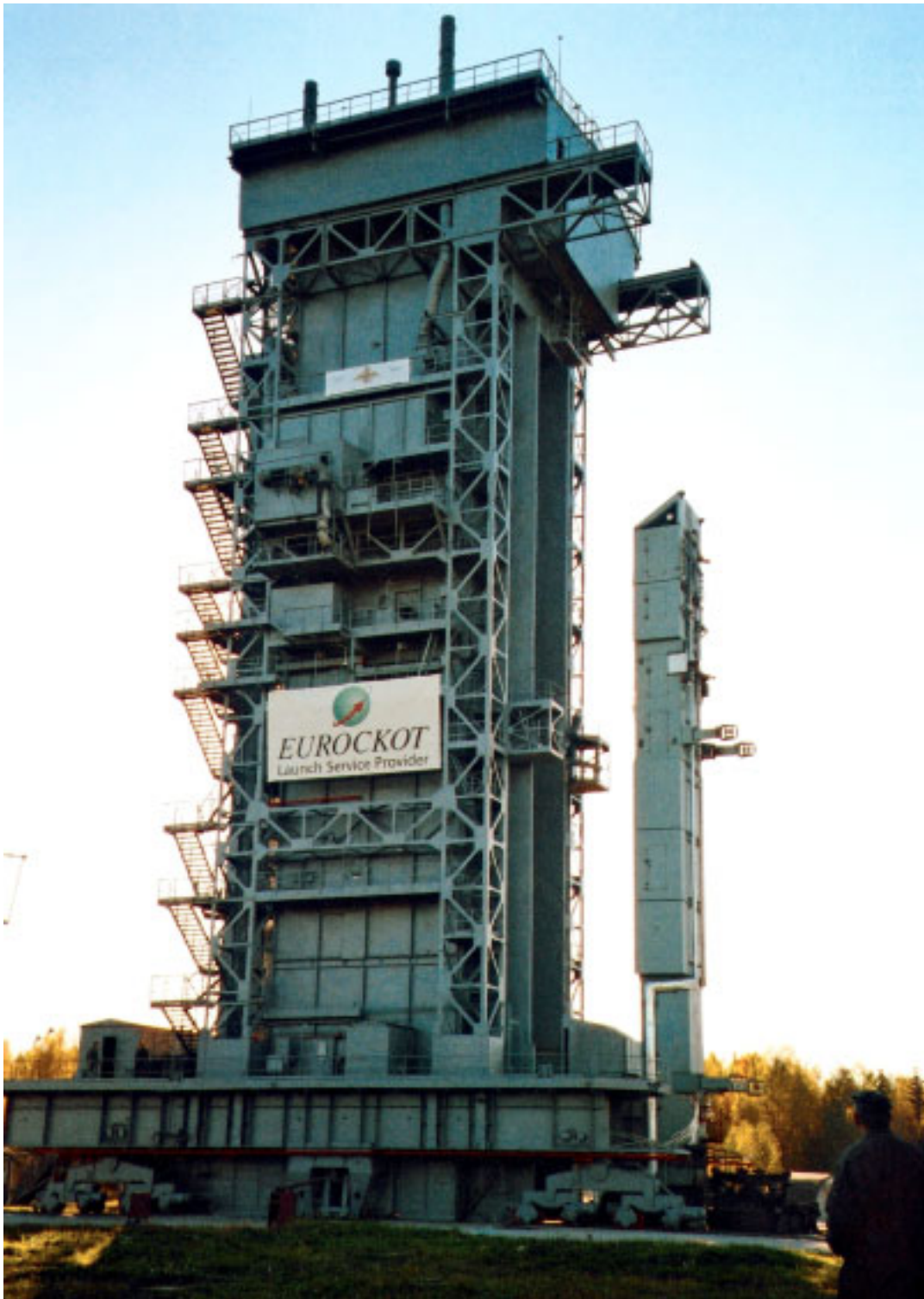
Figure 1-27: Mobile Service Tower and Stationary Column
